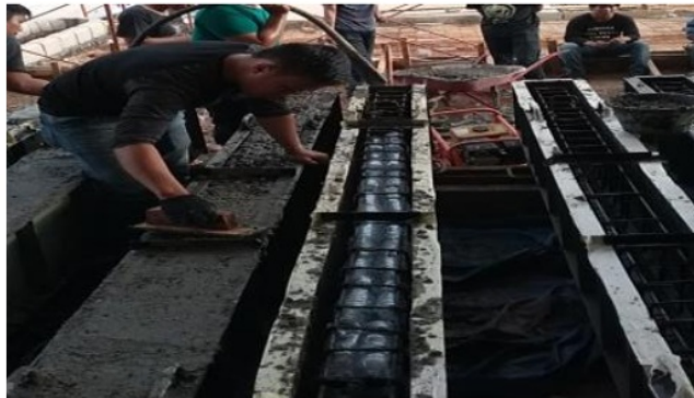
Figure 4. Casting of specimen.
